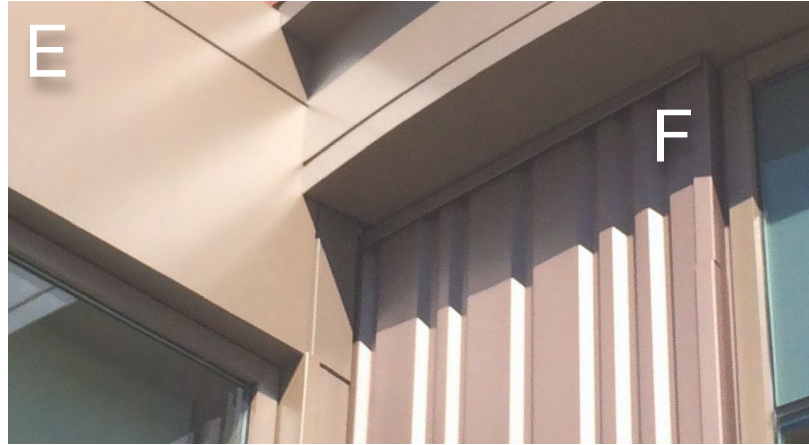
Aluminum Composite Metal Panel (E) | Champagne Rose Single Skin Metal Wall Panel (F) | Champagne Rose
