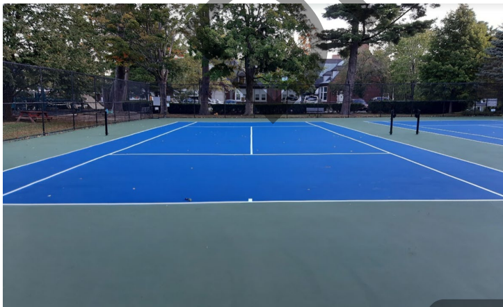
Lower Falls Tennis Courts: resurfacing in progress
