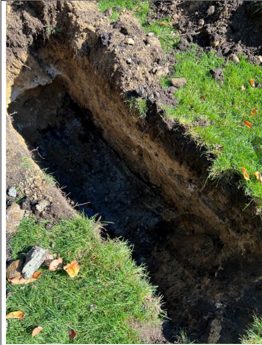
Test Pit TP-1
