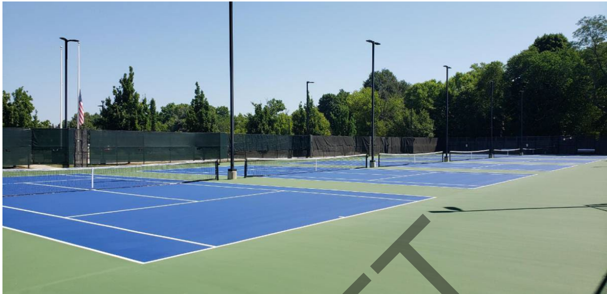
Newton North High School Tennis Courts
