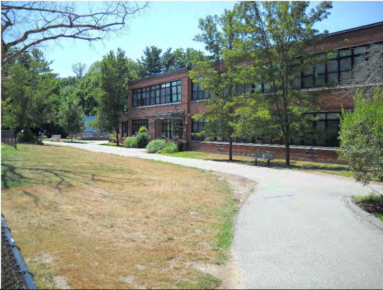
Photo #1: Front view of building.
