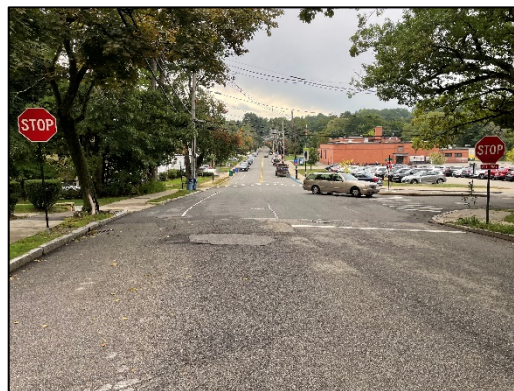
Photo 1: Dedham Street at Walnut Street
