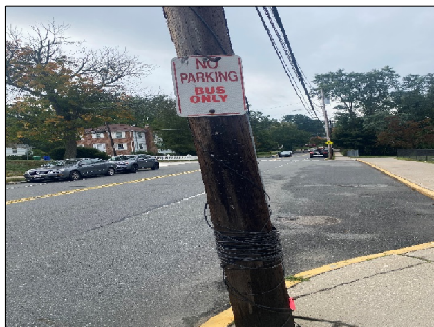
Photo 5: Signage outlining parking restriction for bus pull-off area, with yellow curb striping to further guide buses and restrict passenger cars from using the area.
