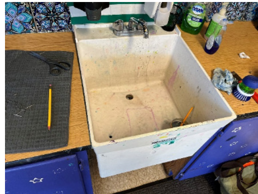
Art Room sink is residential laundry type sink, which is code compliant and functional but an unusual application for an institutional building.
