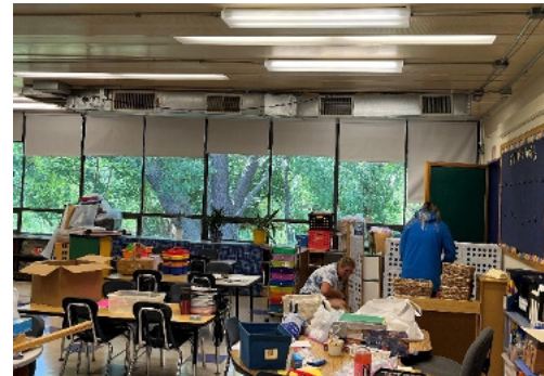
L - Modular annex with end mounted trailer home type AC unit. C - 1958 Annex with gas rooftop provides HVAC for the classrooms. R - Exposed ductwork with no attenuation on return ductwork, resulting in noise level far above what is considered acceptable in today's teaching environment.
