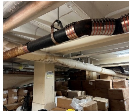
L - Shows original vintage cast iron waste piping in basement with lead / okum packing, showing exterior corrosion. R - Same area shows extensive portion which has been replaced.
