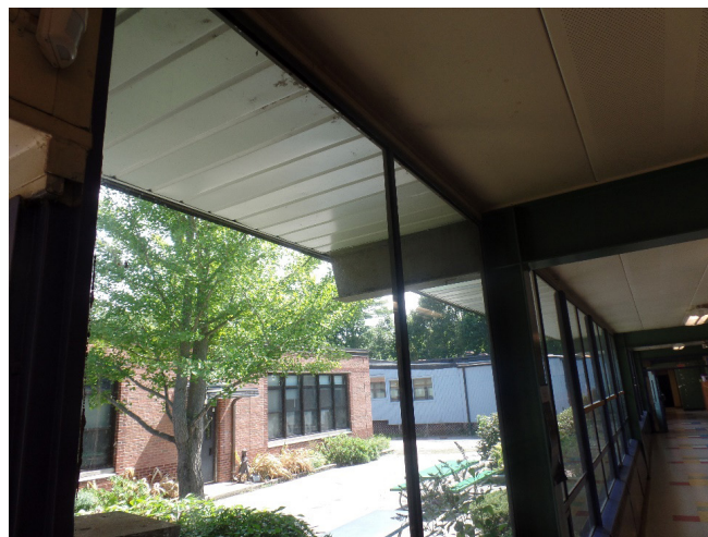
Photo No. 2: 1957 addition roof structure
