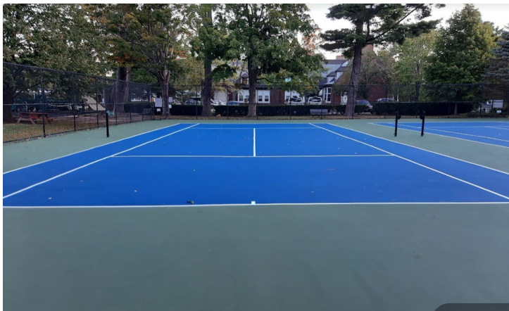
Lower Falls Tennis Courts: resurfacing in progress
