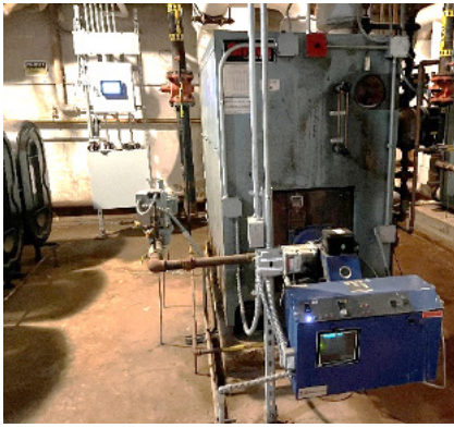
L - Boiler gas piping. C - Recently installed gas fired tank type domestic hot water heater. R - Heater flue.
