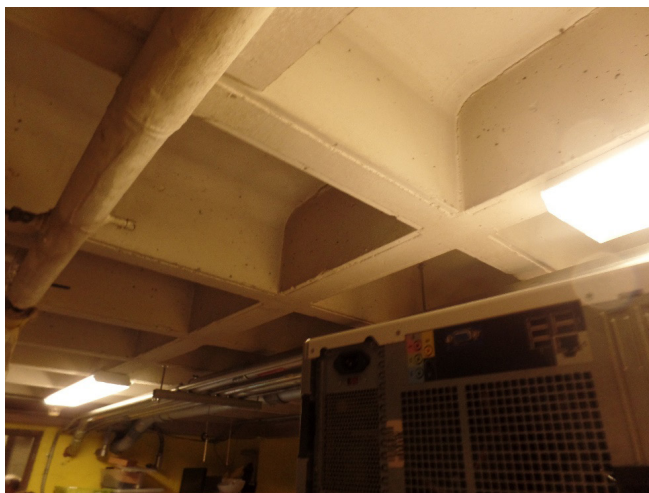
Photo No. 1: Concrete joist first floor slab over basement
