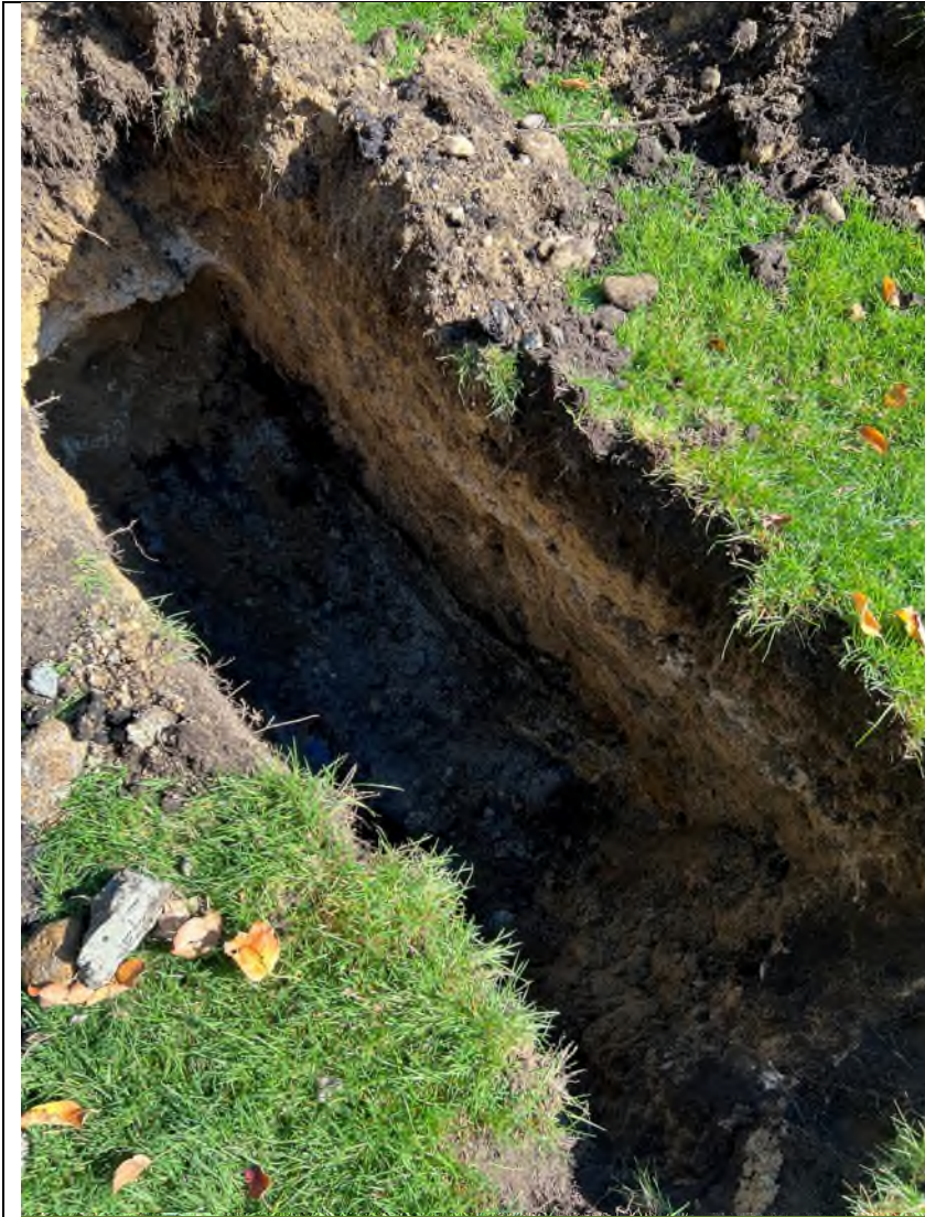
Test Pit TP-1
