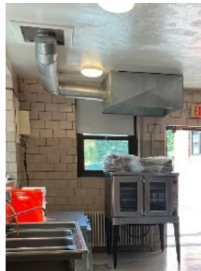
L - Kitchen is limited to preparation and warming functions and without the accommodation for full cooking. C - Hood over a convection oven. R - Hand and pot sinks.
