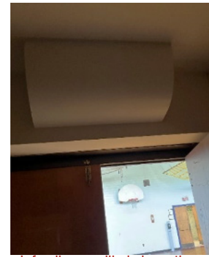
L&C - Gym is heated by steam radiator placed high just below the windows. R - Showing small ventilation ductwork feeding a grill above the storage door.
