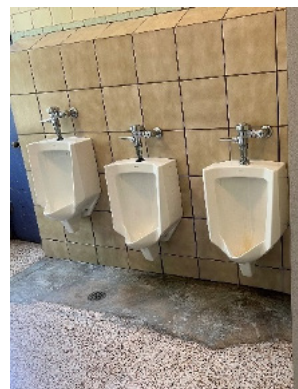
Vitreous china parts of the fixtures in the newer part of the building are original but are in fair condition. Faucets, flushometers and valves have been replaced as needed and are in fair shape.
