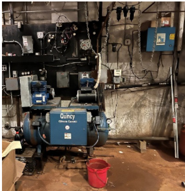
L - Pneumatic control compressor and dryer were in fair working order and are operating. CL - Some spaces were found with two thermostats. CR - Right side thermostat was found to be Johnson Controls pneumatic thermostat; left side thermostat was Delta DDC Controls.
