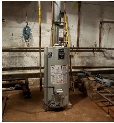
L - Boiler gas piping. C - Recently installed gas fired tank type domestic hot water heater. R - Heater flue.
