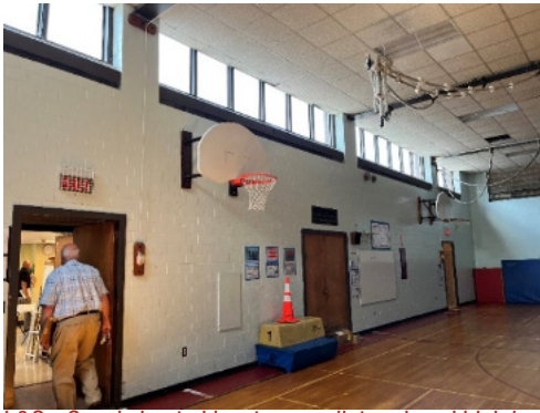
L&C - Gym is heated by steam radiator placed high just below the windows. R - Showing small ventilation ductwork feeding a grill above the storage door.
