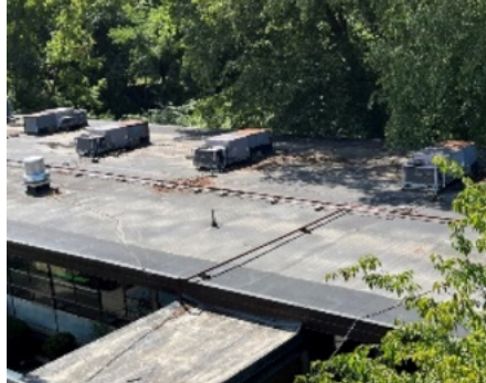
L - Modular annex with end mounted trailer home type AC unit. C - 1958 Annex with gas rooftop provides HVAC for the classrooms. R - Exposed ductwork with no attenuation on return ductwork, resulting in noise level far above what is considered acceptable in today's teaching environment.
