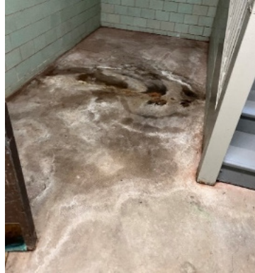
L&C - Chronic flooding of basement level. R - One of numerous sump pumps, which have to be replaced frequently due to its nearly continuous operation.
