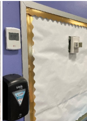
L - Pneumatic control compressor and dryer were in fair working order and are operating. CL - Some spaces were found with two thermostats. CR - Right side thermostat was found to be Johnson Controls pneumatic thermostat; left side thermostat was Delta DDC Controls.
