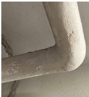
Potential ACM encapsulation was observed at pipe fitting insulation.
