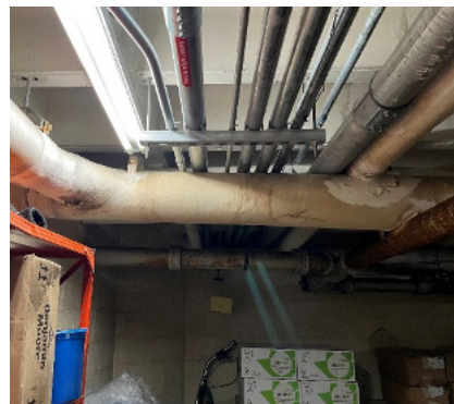
Potential ACM encapsulation was observed at pipe fitting insulation.
