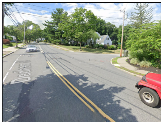
Photo 2: Dedham Street at Bound Brook Road
