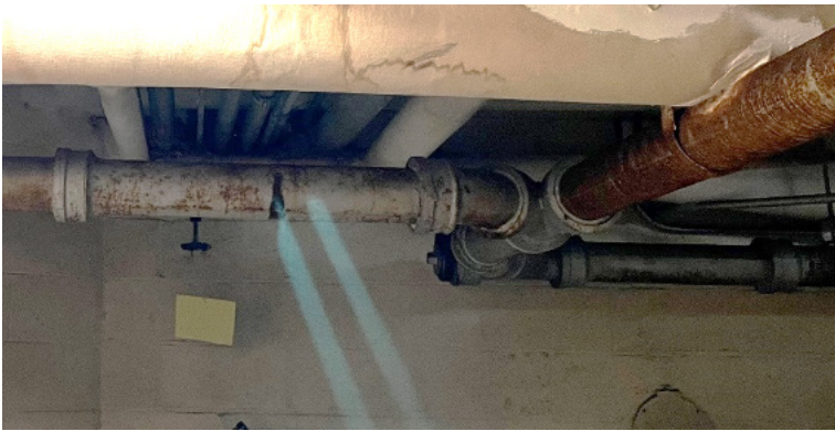
L - Shows original vintage cast iron waste piping in basement with lead / okum packing, showing exterior corrosion. R - Same area shows extensive portion which has been replaced.
