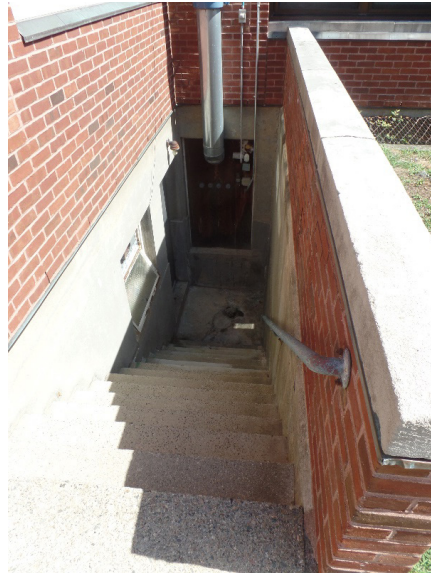
Photo No. 8: Exterior stair to 1951 boiler room
