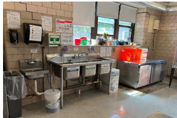
L - Kitchen is not a full cooking type but just a warm-up and preparation type. R - Note that section of hand sink waste piping has been replaced with non-compliant PVC piping; grease interceptor could not be located.
