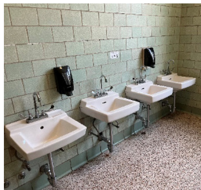
Vitreous china parts of the fixtures in the newer part of the building are original but are in fair condition. Faucets, flushometers and valves have been replaced as needed and are in fair shape.
