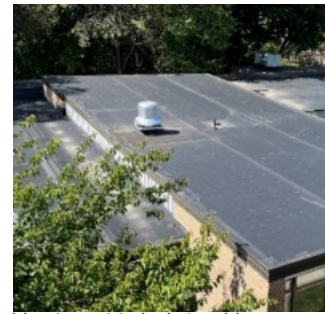
Typical classrooms are heated and ventilated by unit ventilators (L & CL) and wall exhaust (CR), which would not meet today's teaching environment acoustical requirements. R - Central roof exhaust fan assure
