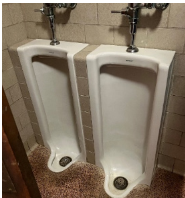
L - Urinals in the older part of the building are not code compliant. All - Vitreous china parts of the fixtures are original but are in fair condition. Faucets, flushometers and valves have been replaced as needed and are in fair shape.
