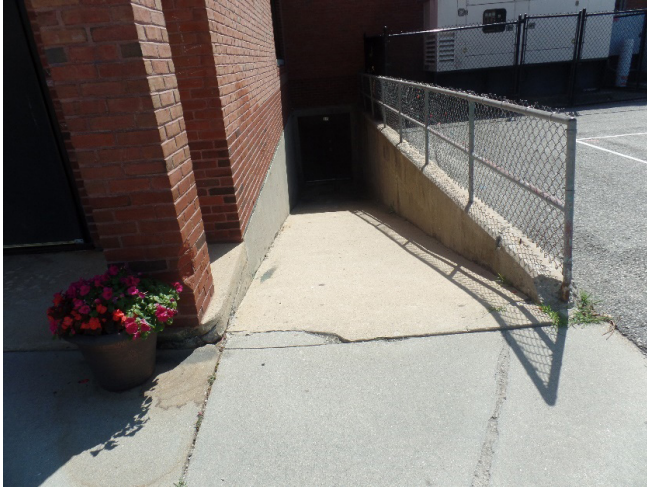
Photo No. 7: Exterior ramp to 1951 basement
