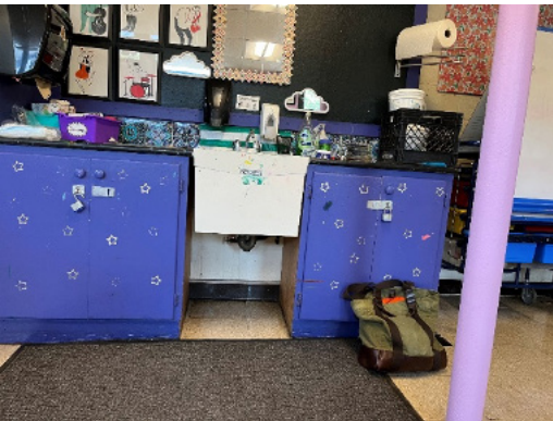
Art Room sink is residential laundry type sink, which is code compliant and functional but an unusual application for an institutional building.
