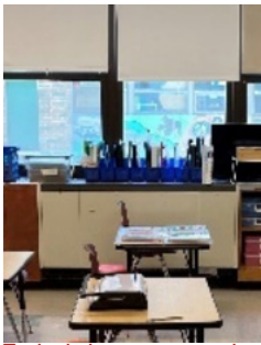
Typical classrooms are heated and ventilated by unit ventilators (L & CL) and wall exhaust (CR), which would not meet today's teaching environment acoustical requirements. R - Central roof exhaust fan assure
