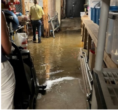
L&C - Chronic flooding of basement level. R - One of numerous sump pumps, which have to be replaced frequently due to its nearly continuous operation.
