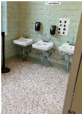
Vitreous china parts of the fixtures in the newer part of the building are original but are in fair condition. Faucets, flushometers and valves have been replaced as needed and are in fair shape.
